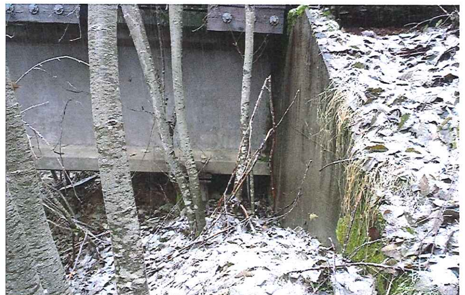
CK2248 Left Abutment
