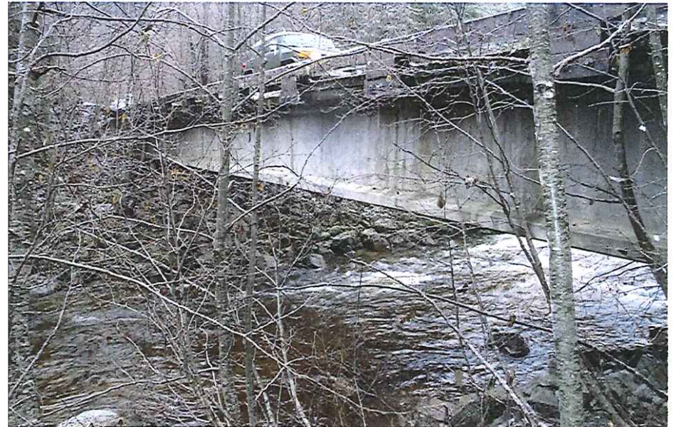
CK2248 From Downstream
