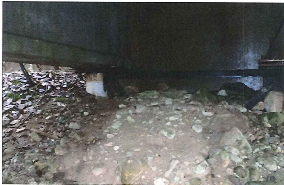
CK2248 Left Abutment Bearing
