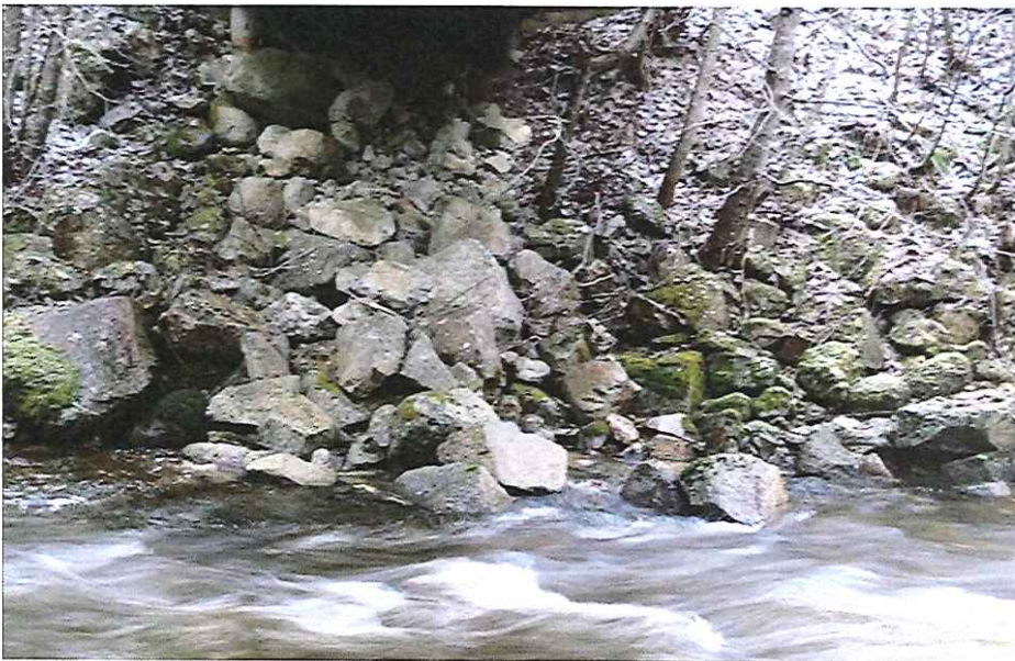
CK2248 Right Abutment
