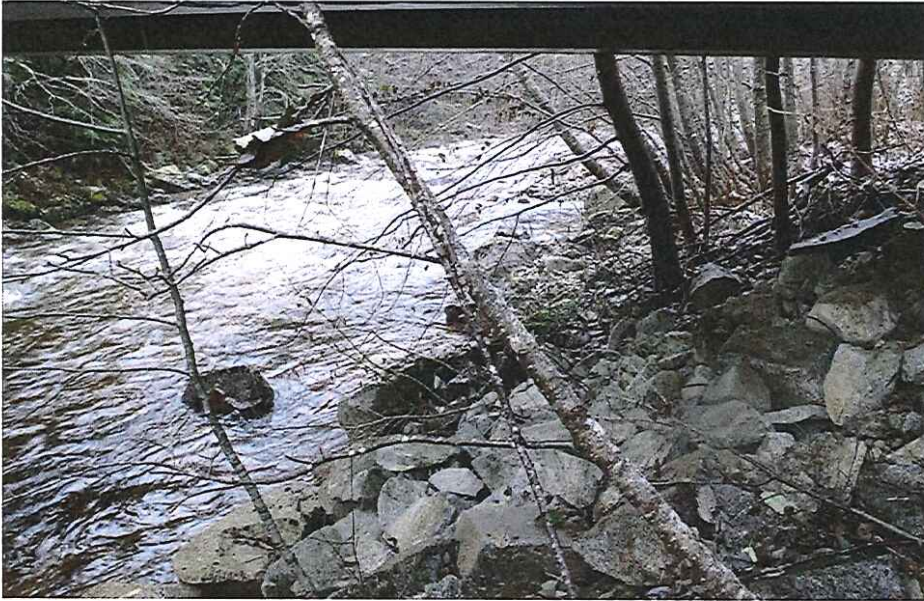
CK2248 Left Abutment Rip Rap
